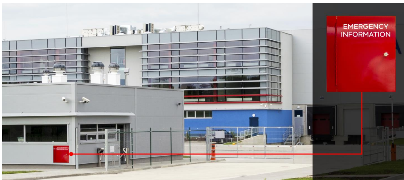
Figure 22: the Emergency Information Container (EIC) should be located at your site as close as practical to all vehicle entrance(s).
